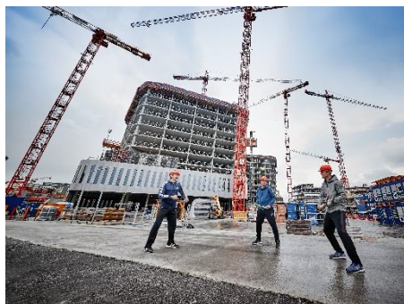
To the top WOLFFKRAN: Professional young talents Cedrik-Marcel Stebe, Maximilian Marterer und Kevin Krawietz (from left to right) of the TennisBase Oberhaching in front of WOLFF cranes used by PORR Germany for the Bavaria Towers construction project.
